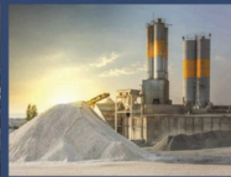
CONCRETE BATCHING PLANTS
